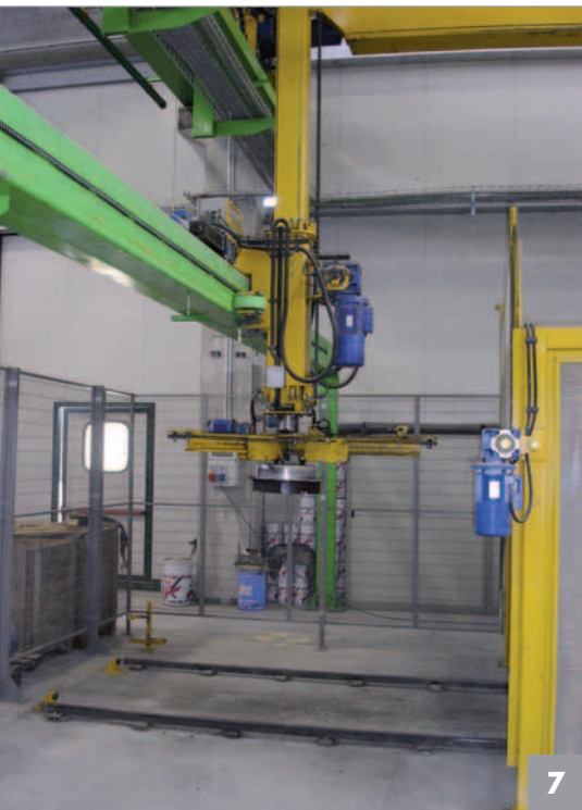
Steel pallet handling
