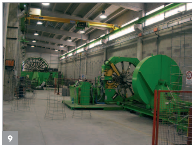
Production of reinforcement cages
